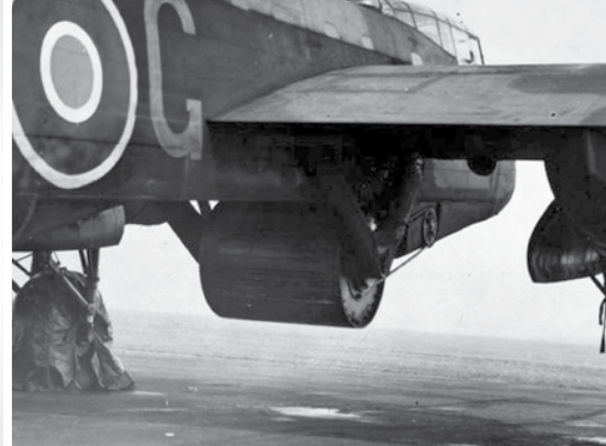
The "bouncing bomb" code-named "Upkeep" and the attachment system. Note the chain drive that spun up the bomb to 400 rpm to ensure that the bomb skipped across the water. RAF/BOMBER COMMAND MUSEUM
